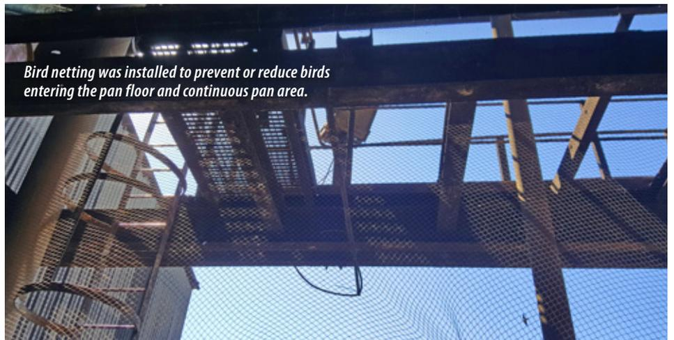
Bird netting was installed to prevent or reduce birds entering the pan floor and continuous pan area.
