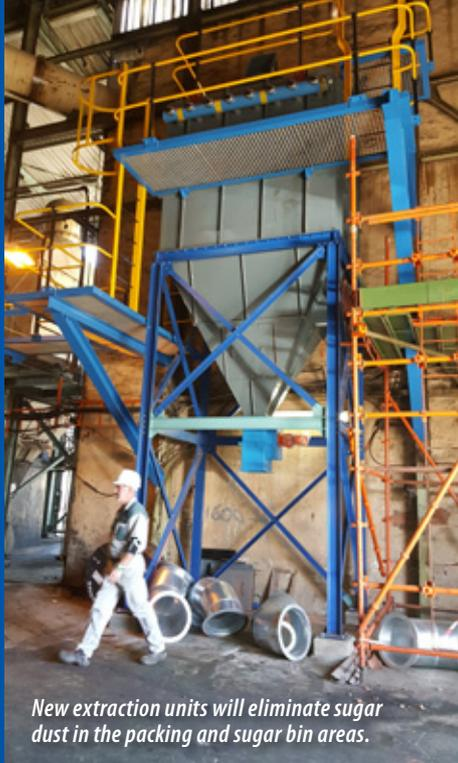
New extraction units will eliminate sugar dust in the packing and sugar bin areas.
